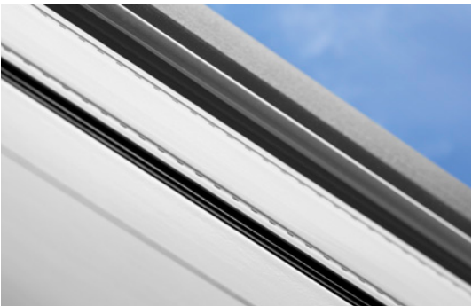
Connection between sash, glazing and outside cladding.
